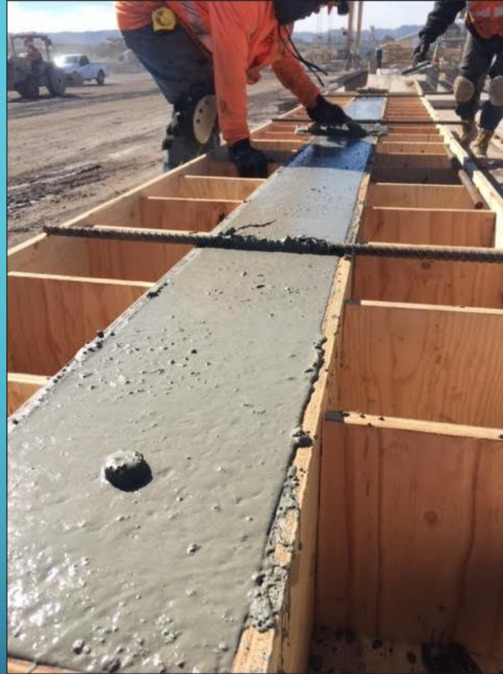
Figure 11 Screeding of Concrete [2]
