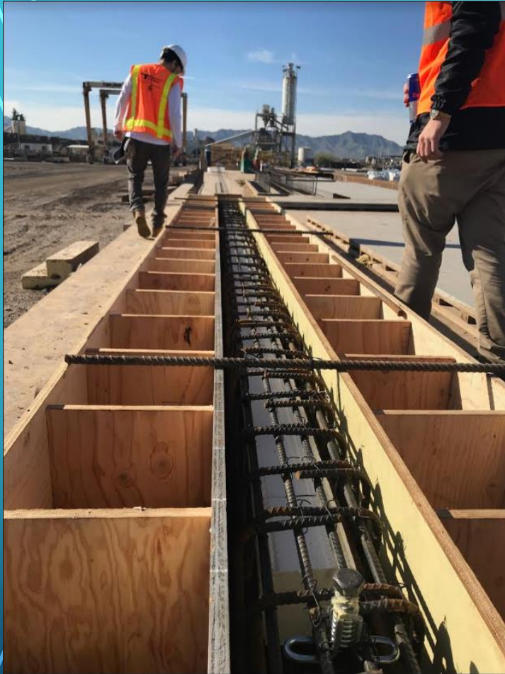
Figure 10 Formwork [2]
